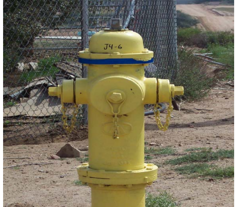
This hydrant is approved for all residential and light commercial applications. Fire Flow letter shall be submitted with application. This type shall be installed for all new applications
